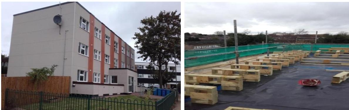
This was a £625,000 Innovate UK funded trial involved upgrading a block of six flats to EnerPHit standard by way of an innovative Off-site Wrap-around Large Scale (OWLS) retro-fit. The residents remained in situ throughout the work, so minimising disruption to their lives, before they were left to enjoy all of the benefits associated with Passivhaus. Our partners in the project included Beattie Passive, Encraft, Solihull Community Housing and Coventry University.
