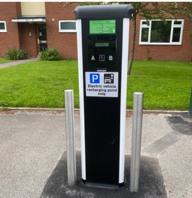
One of the EV charging bays
