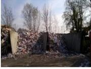
Recycling which is collected is taken to Bickenhill Household Waste Recycling Centre where it is deposited into bulking bays. There are two bays - one for glass and one for mixed recycling . The mixed recycling is transported by articulated lorry to the MRF.
