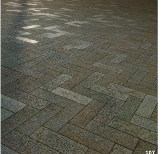
Granite aggregate concrete paving
