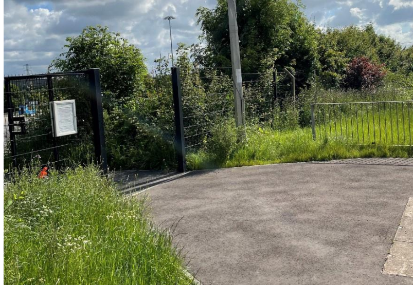
Photograph showing footpath closed (right) and new entryway / path (left)
