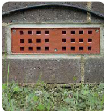
Automatic / Self closing air brick
