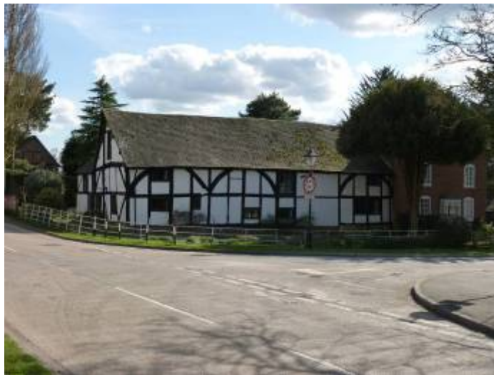
Timber framing at The Malt House
