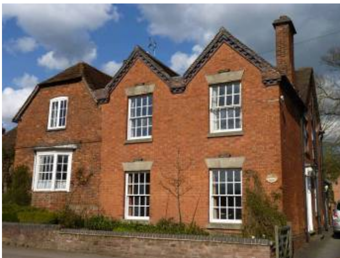
The Forge and Butchers House, 'positive' buildings on Spencer's Lane
