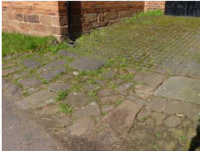
Survival of sandstone paving and stable setts outside the former smithy at The Forge
