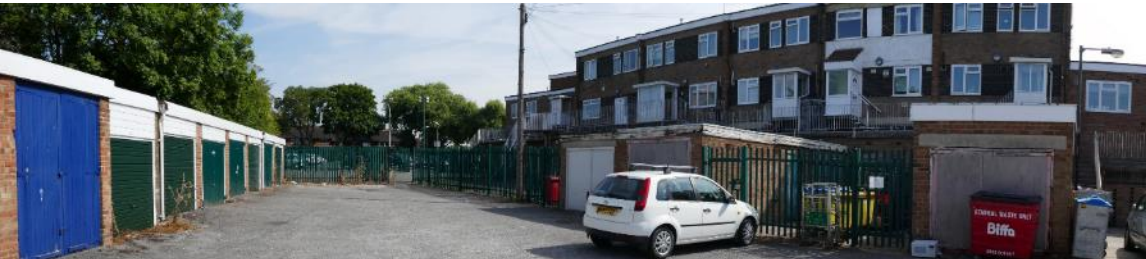
Rear garages, service yard and access to upper floor residential units
