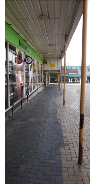
Retail precinct and canopy
