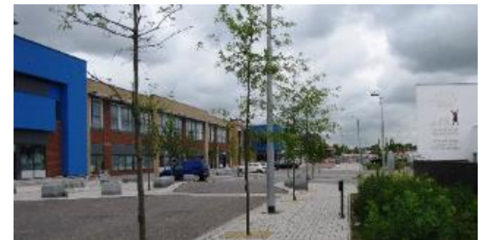
Smiths Wood Local Centre before and after intervention
