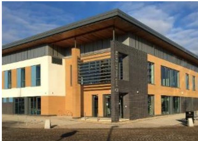
Chelmund's Cross Local Centre during construction and after completion
