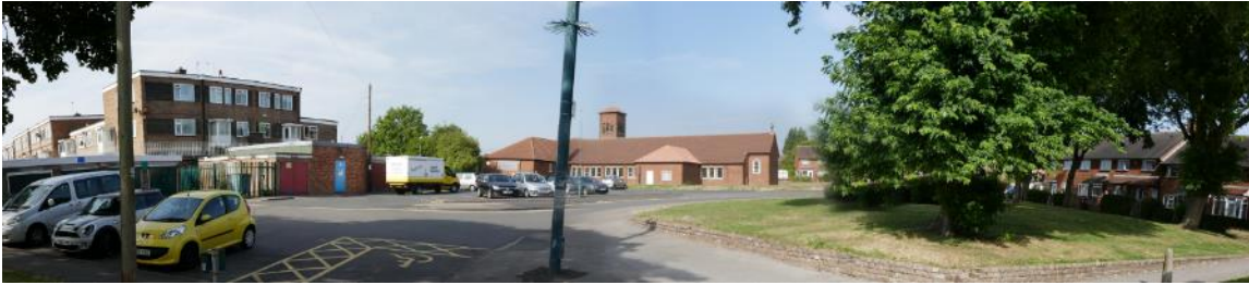
St Barnabas Church and rear of the retail precinct and residential units from Colling Walk
